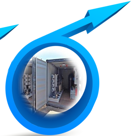
Hsinchu Emergency Desalination Units 13,000 ton/day
